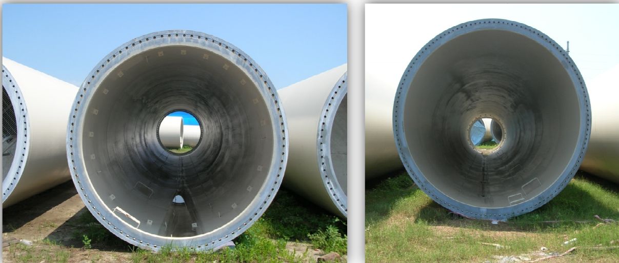
In April 2005, the interior of 22 wind mills have been treated with the system ZINGA 1 x 60 µm DFT + Zingaceram ZM EP TOP 2 x 100 µm DFT.
